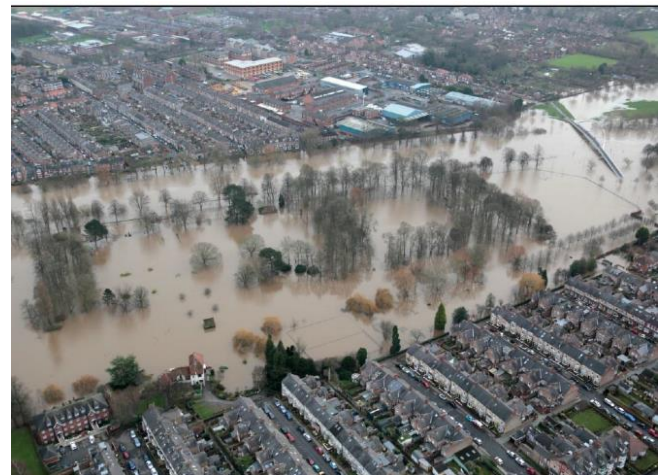
Flooding by Rowntree Park and Millennium Bridge
